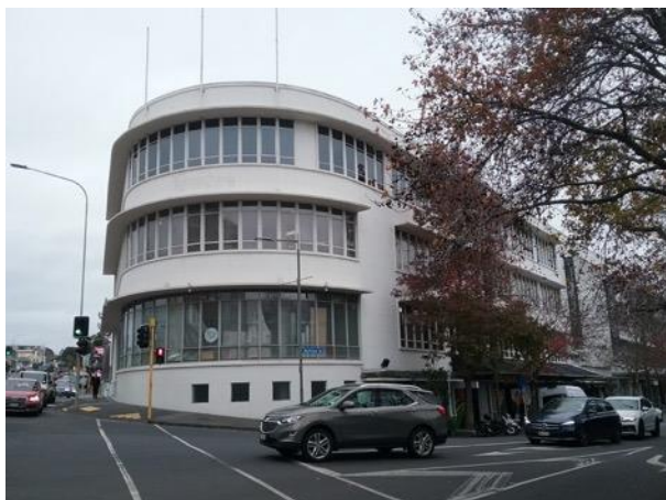
Figure 5: Auckland Electric Power Board office building, 2-38 Nuffield Street
