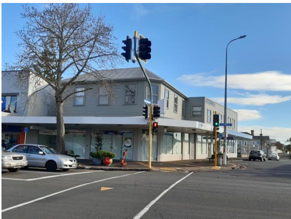
Figure 11: Arch Hill Hotel (former), 584 Great North Road
