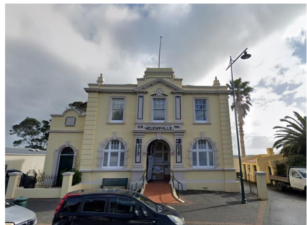
Figure 4: Helensville Post Office, 102 Commercial Road (Google Street View, July 2020)
