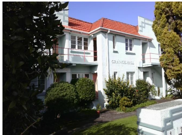
Figure 4: Grange Hall Apartments, 492 Mount Eden Road
