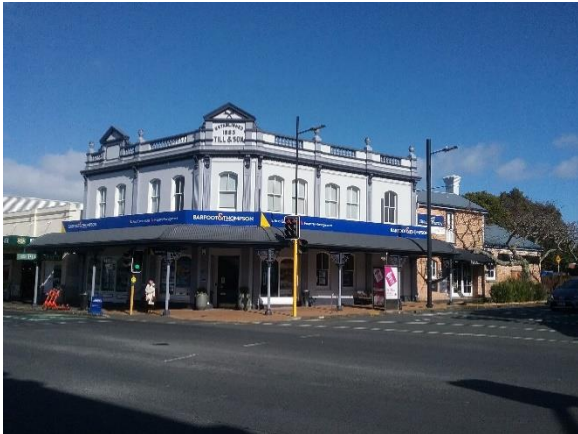
Figure 1: Till and Son Building, 427-429 Mount Eden Road
