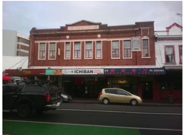
Figure 2: Kents Buildings, 481-487 Khyber Pass Road
