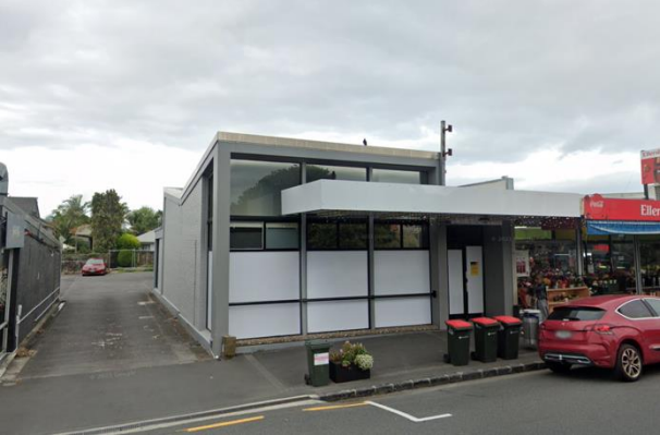
Figure 7: 133A Main Highway (Google Street View, March 2021)
