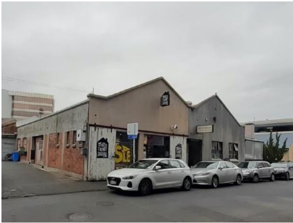
Figure 7: 2-8 Osborne Street (3 York Street)
