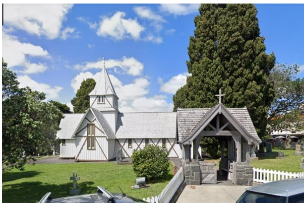
Figure 3: All Saints Church, 9 Selwyn Road (Google Street View, November 2020)
