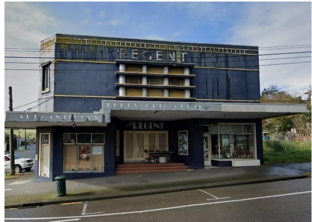
Figure 2: Regent Theatre, 14 Garfield Road (Google Street View, July 2020)
