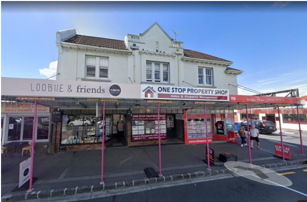
Figure 5: Mackenzie's Buildings, 114-116 Main Highway (Google Street View, March 2021)
