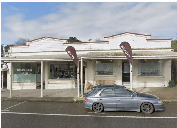
Figure 3: Cameron Shops, 81 Commercial Road (Google Street View, July 2020)
