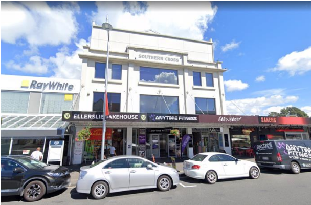
Figure 6: Southern Cross Building, 87-93 Main Highway (Google Street View, March 2021)
