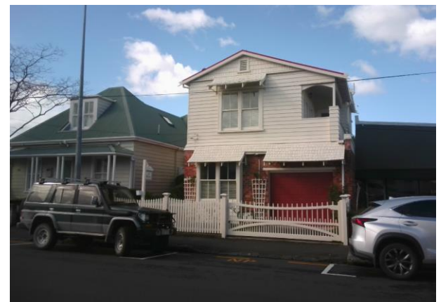
Figure 6: 14 and 16 Wynyard Street
