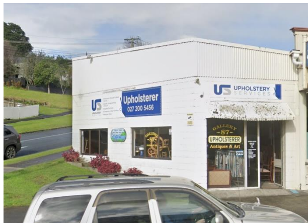
Figure 12: 87 Commercial Road (Google Street View, July 2020)
