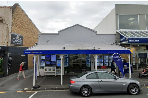
Figure 4: Former Snooker Saloon, 107-109 Main Highway (Google Street View, March 2021)
