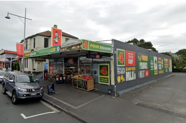
Figure 9: Four Square, 126 Main Highway (Google Street View, March 2021)
