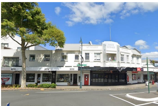
Figure 1: McInness Building, 127 Picton Street (Google Street View, November 2020)
