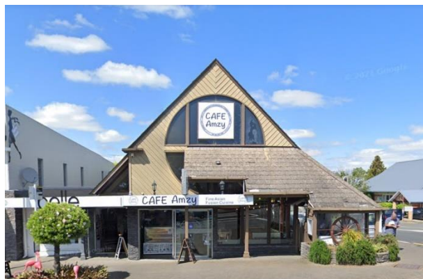
Figure 9: 21 Picton Street (Google Street View, November 2020)
