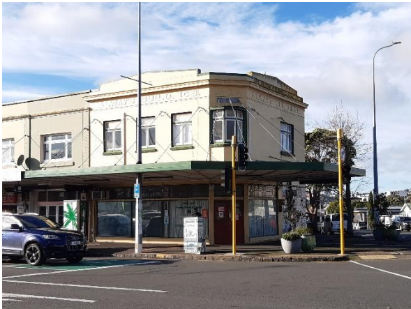
Figure 1: Alway's Buildings, 543 Great North Road
