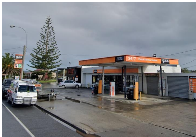
Figure 11: 4-16 Railway Street (Google Street View, July 2020)
